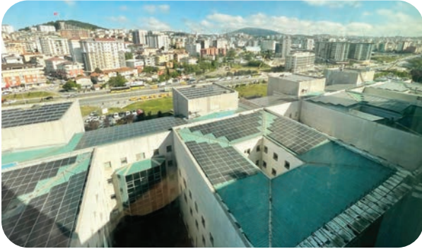
İstanbul Pendik Hospital / 500 kW
