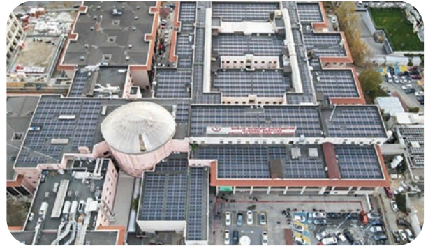
İstanbul Bağcılar Hospital / 800 kW
